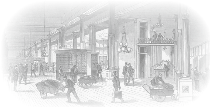
Interior of view of the New York Post Office
